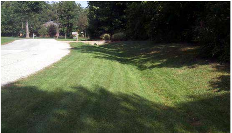
Grassed swale - directs stormwater from street to water trees
