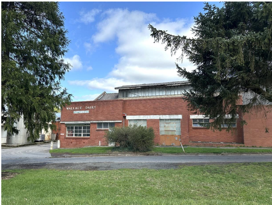
Building 1: Former Butter Factory
