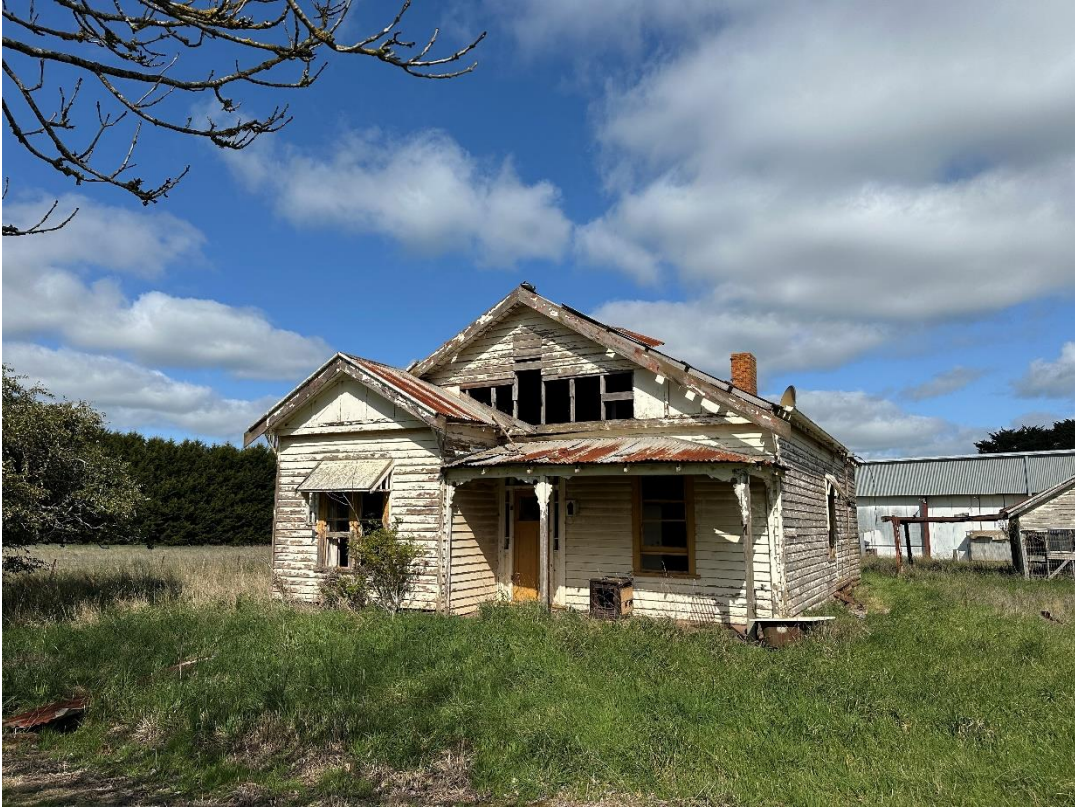
Building 6: Timber interwar Bungalow
