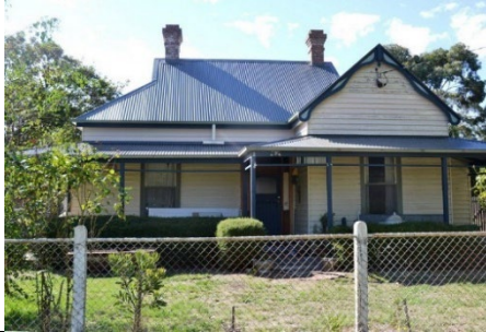
Photo 2: 18 Duncan Street, Ballan, 2014. Source: David Rowe..
