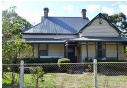
Photo 4: 18 Duncan Street, Ballan, 2014. Source: David Rowe.
