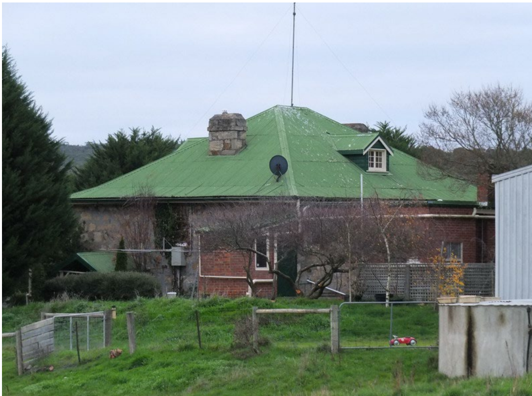
Photo 4: Hunterston, rear/side view from Ballan-Egerton Road, 2014. The cellar entrance (gabled roof) is shown below the main roof line.
