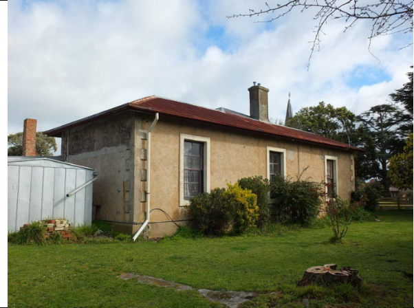
Photo 7: Former St. Paul's Manse, side (east) elevation, 2014.
