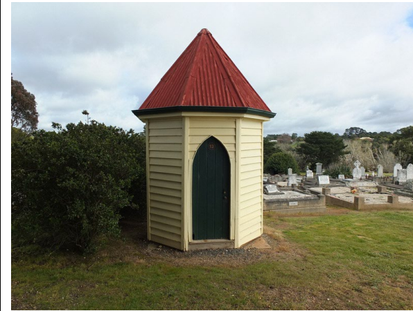
Photo 9: Former Robing Room, near main entrance, 2014.
