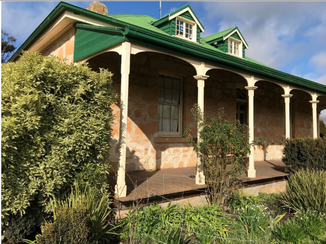
Photo 5: Hunterston, detail of front elevation, 2020
