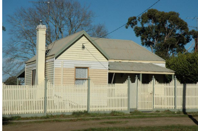
Photo 2: Dwelling in 2009, undergoing repairs
