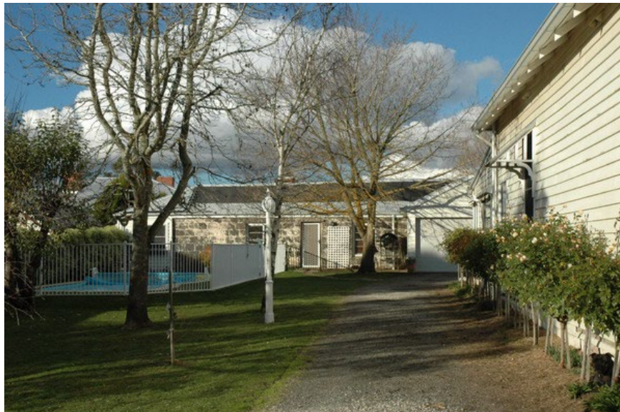
Photo 2: Former stone bake house (background), as viewed from outside the property in Fisken Street, 2009.
