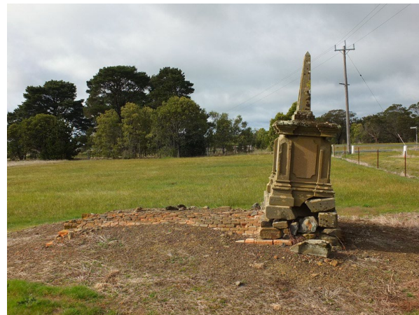
Photo 3: Side view of the vault of Thomas Henry Pyke, showing significant lean of the pedestal and obelisk, and substantially deteriorated base, 2009.
