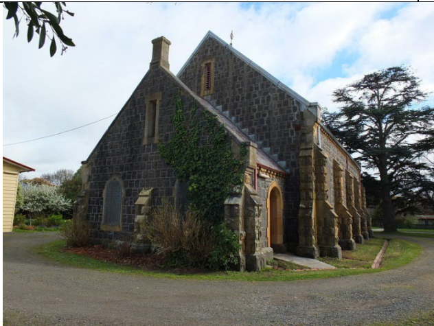
Photo 5: St. Paul's Church, rear (south) elevation, 2014.
