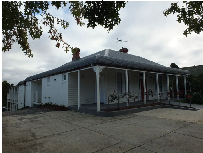
Photo 5: Lea Hurst, 2015, showing introduced return bullnosed verandah and addition on west side.
