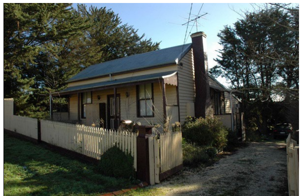
Photo 3: Dwelling, 56 Inglis Street, 2009, prior to the construction of the garage.
