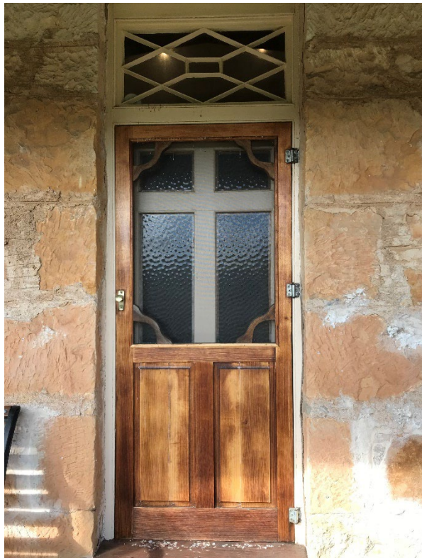
Photo 2: Hunterston, showing front door and original timber framed transom, 2020.
