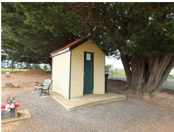
Photo 10: Former Sexton's building, near main entrance, 2014.
