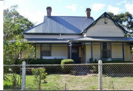
Photo 5: 18 Duncan Street, Ballan, 2014. Source: David Rowe.
