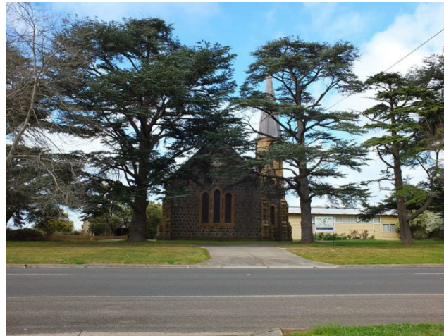
Photo 2: Front setting of St. Paul's Church, showing mature trees and large open spaces each side of the church, 2014.
