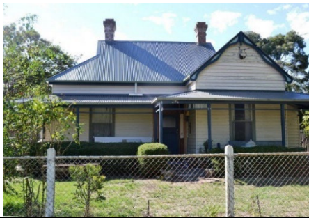
Photo 5: 18 Duncan Street, Ballan, 2014. Source: David Rowe.
