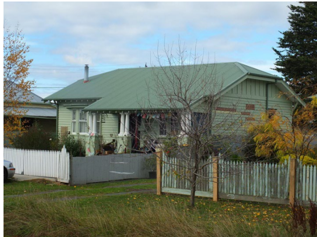
Photo 2: State Saving Bank dwelling, 49 Edols Street, 2014.
