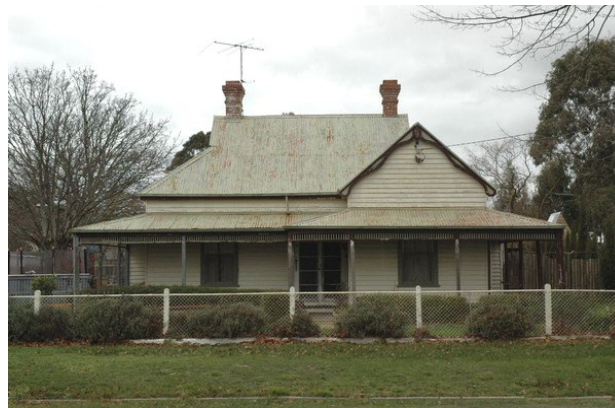
Photo 2: Dwelling, 18 Duncan Street, 2009, showing front double door opening and early timber framed fretwork valance.
