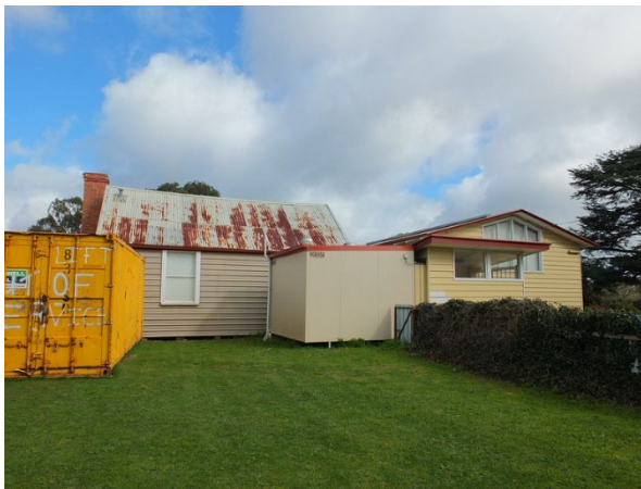
Photo 8: Robertson Memorial Hall, side (east elevation), with postwar hall shown on the right, 2014.
