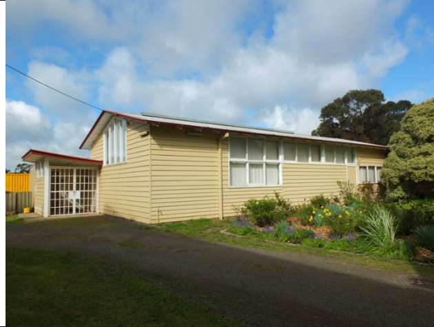
Photo 10: Postwar Sunday School Hall, front (north) elevation, 2014.
