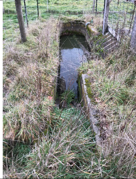
Photo 12: Llandeilo, concrete sheep dip to rear of Shearing Shed, 2020
