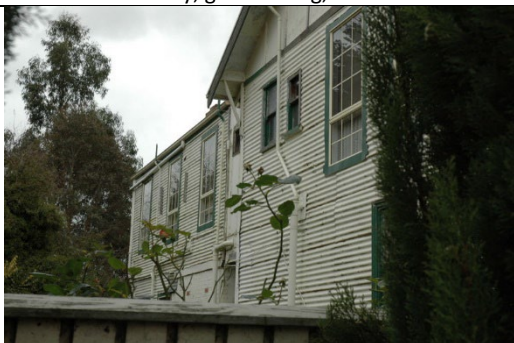
Photo 4: Ballan Hotel, detail of west elevation showing early corrugated galvanised steel roof cladding, 2009.
