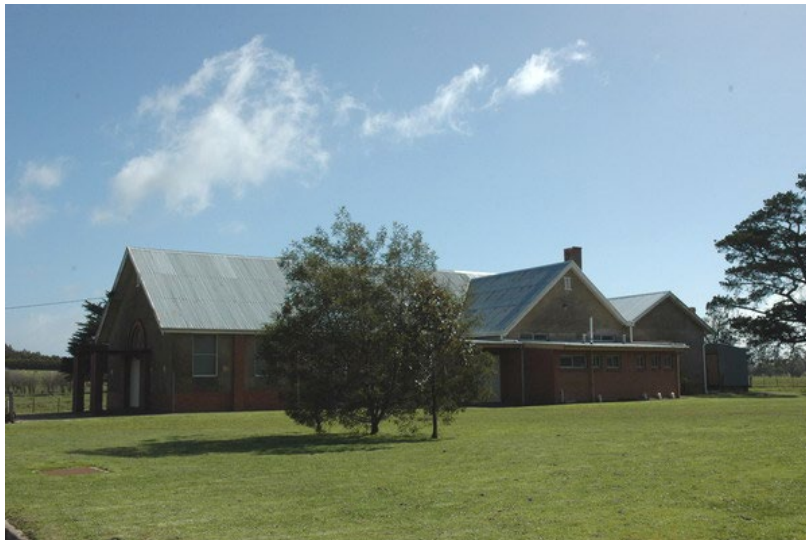
Photo 2: Bungaree Mechanics' Institute & Free Library, east elevation, 2009.
