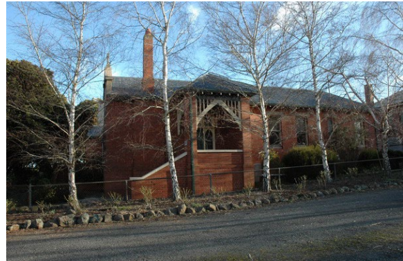
Photo 7: Former St. Michael's Presbytery, north elevation, 2009.
