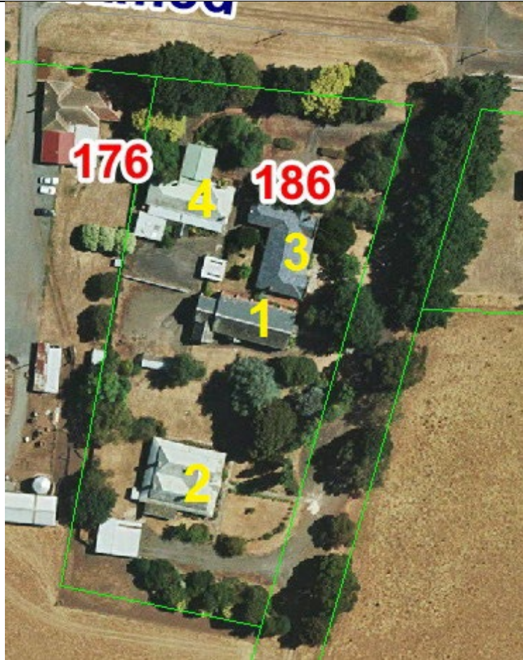
Photo 2: Aerial View of St. Michael's Catholic Church complex.
