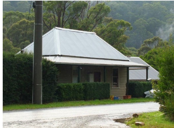
Photo 5: Dwelling, 111 Golden Point Road, Blackwood, 2014. Source: David Rowe.
