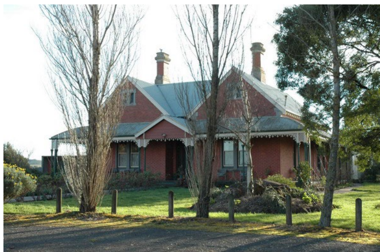
Photo 5: St. Michael's Presbytery, east elevation, 2009.
