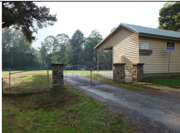
Photo 7: Random rubble gate piers and metal gates, 2014.
