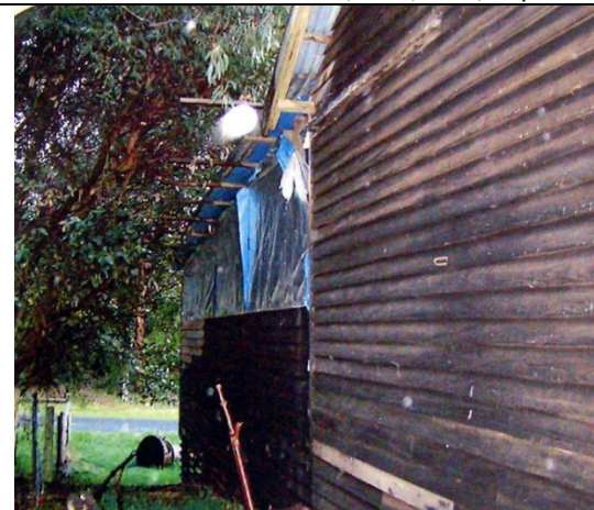
Photo 7: Former Police Stables showing skillion addition under construction, n.d. [c.1978].
