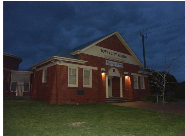
Photo 9: Former Town and City Mission building, Ballarat.
