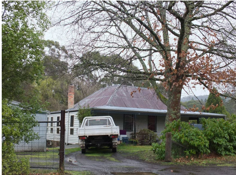
Photo 2: Dwelling, 4 Albert Street, Blackwood front (east) and south elevations, 2015.
