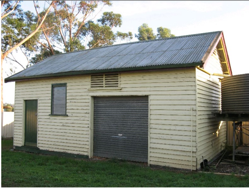
Photo 9: Dartmoor Police Stables, 19-23 Wapling Street, Dartmoor, 2009.
