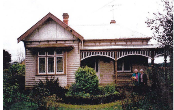
Photo 5: Sunny Rise, front (south) elevation, 2010. Source: Dennis Speilvogel.
