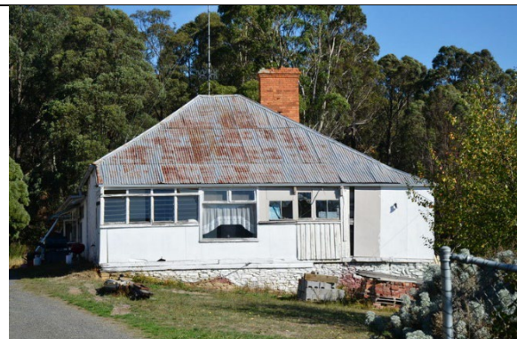
Photo 8: Dwelling, 6 Terrill Street, Blackwood 2014.
