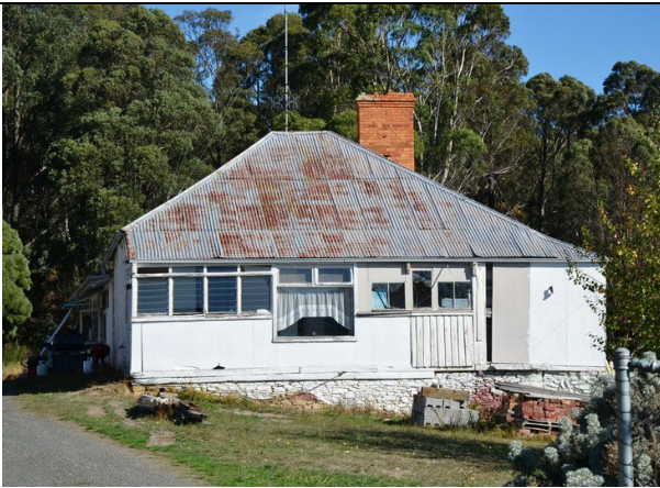
Photo 4: Dwelling from Terrill Street (east elevation), 2014.
