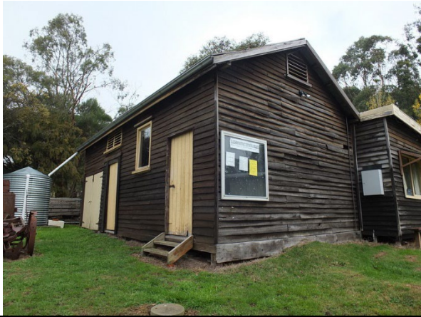
Photo 2: Former Police Stables, 2014.
