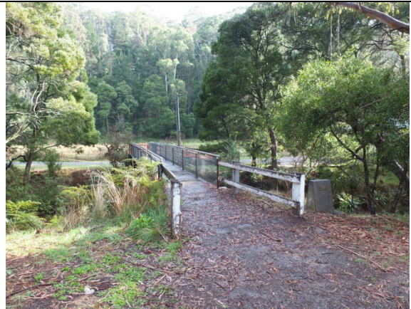
Photo 12: W.A. Matheson Bridge, looking north, 2014.
