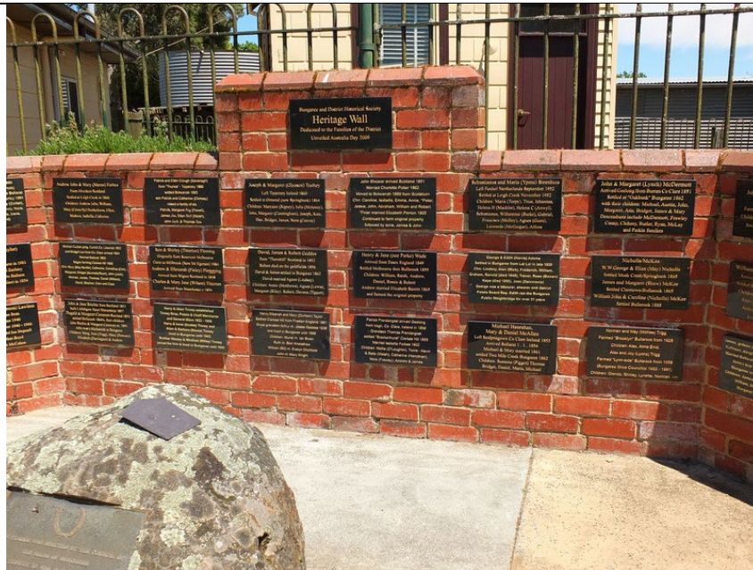
Photo 2: Portion of commemorative wall with boulder in front, 2014.
