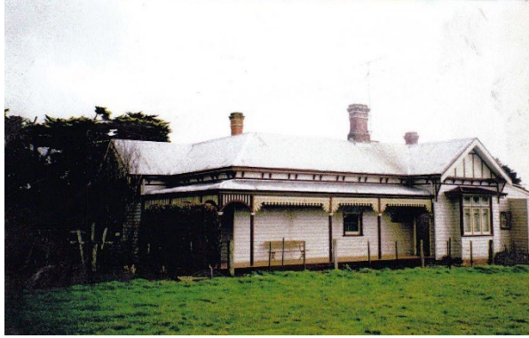
Photo 4: Sunny Rise, east and front (south) elevations, 2010. Source: Dennis Speilvogel.
