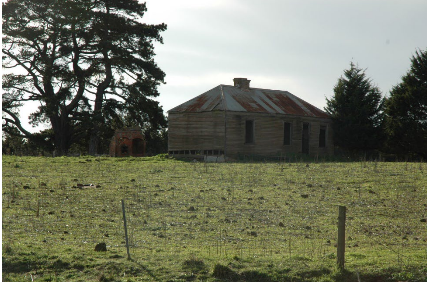
Photo 3: Original homestead further south, as viewed from Torpys Road, 2009.
