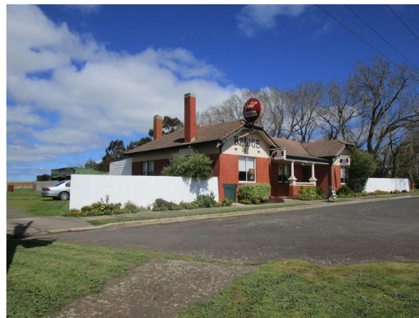
Photo 4: Bridge Hotel showing front & east elevations, 2016.
