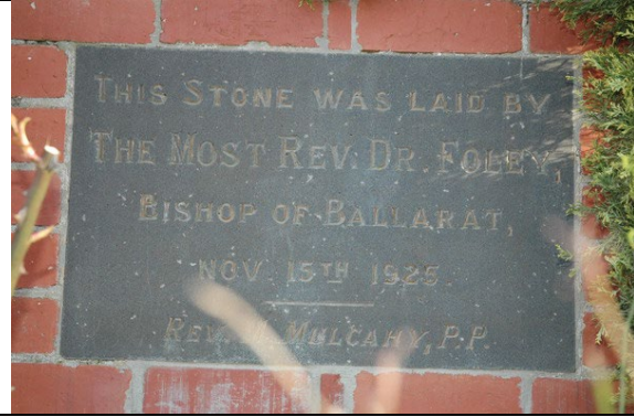
Photo 9: Former St. Michael's School, foundation stone, north elevation, 2009.
