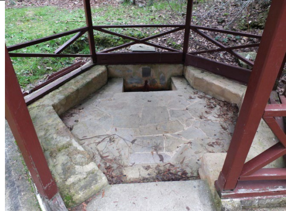
Photo 5: South pavilion showing water outlet pit, 2014.
