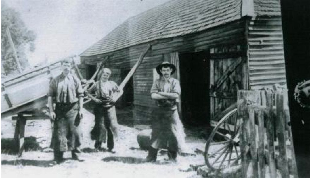
Photo 3: Devereux's blacksmith's shop, n.d. Source: Bungaree & District Historical Society.
