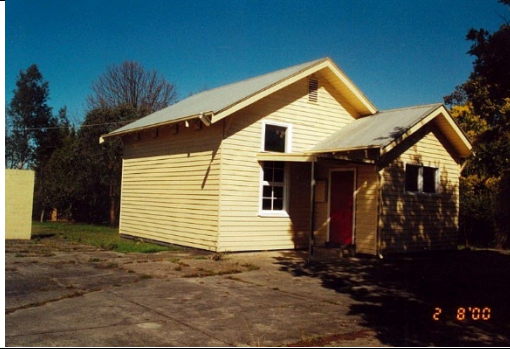
Photo 7: Former Leongatha State School No. 3251, 7975 Bass Highway, Leongatha South, 2000. Source: Hermes.
