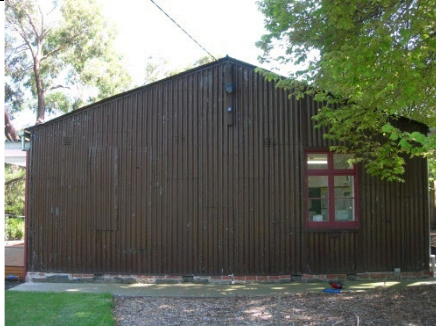
Photo 12: Walmsley House, 1 Gatehouse Street, Parkville, 2008. Source: SOHE
