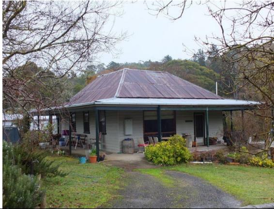
Photo 4: Dwelling, 4 Albert Street, Blackwood, 2014. Source: David Rowe.
