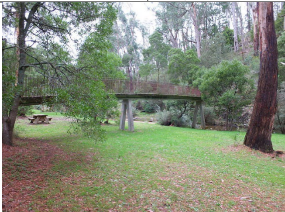
Photo 6: Concrete bridge spanning the Lerderderg River, 2014.
