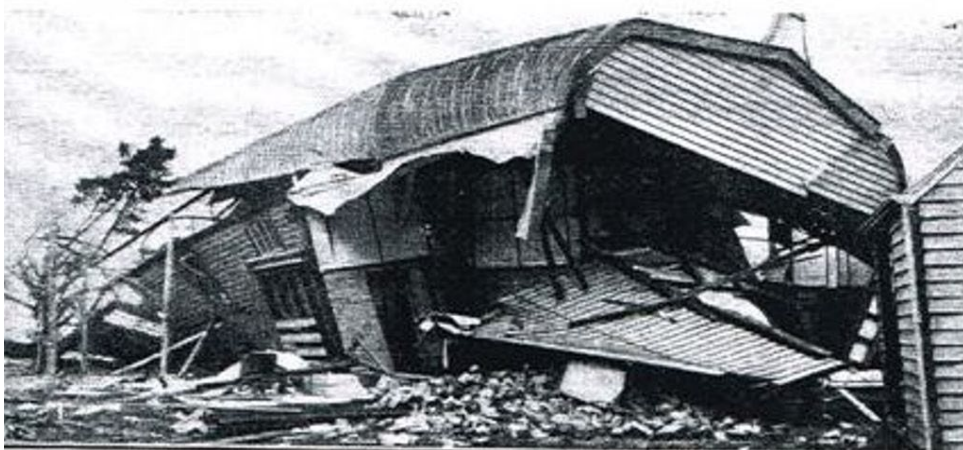
Photo 9: Mechanics' Institute, Bungaree Wallace Road, 1927, substantially damaged by a cyclone.
