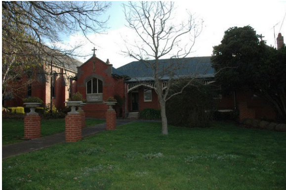
Photo 6: Former St. Michael's Presbytery, east elevation, 2009.
