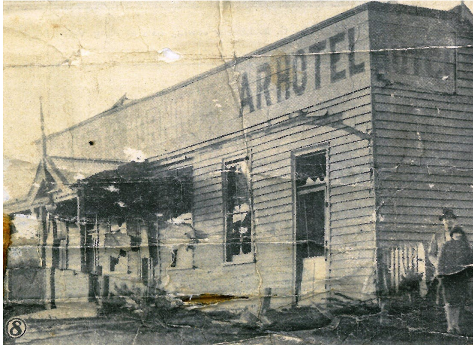
Photo 4: Substantially damaged Morning Star Hotel caused by the cyclone, 1927.
