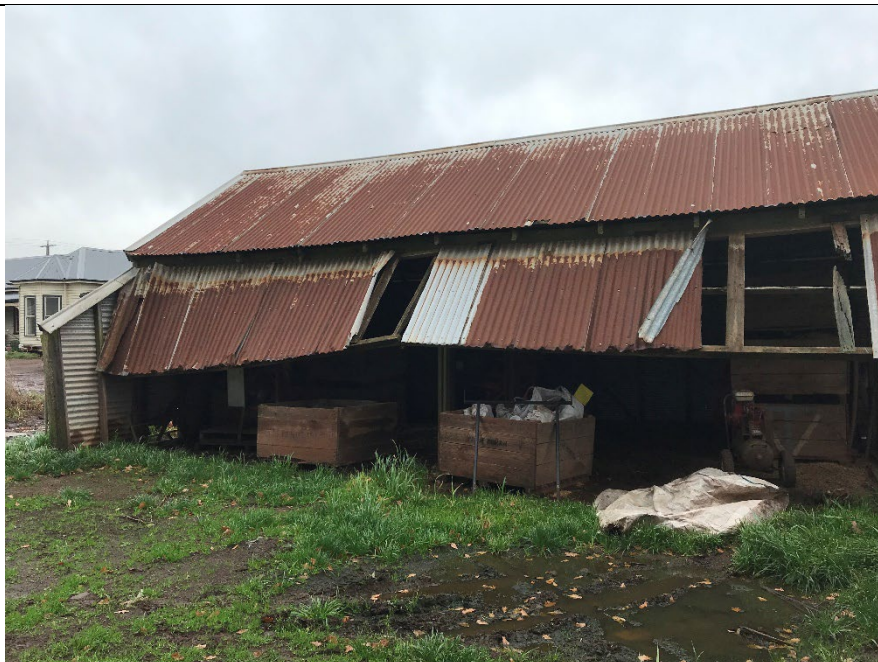
Photo 5: Outbuilding - The Big Shed, Hawthorn Farm, Bungaree, 2020
