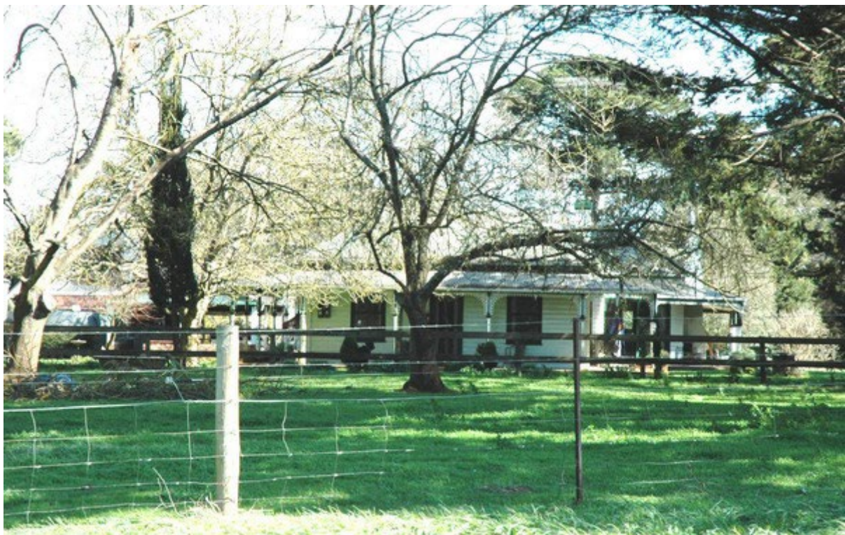
Photo 2: Mayfield, front façade from Lesters Road, 2009.
