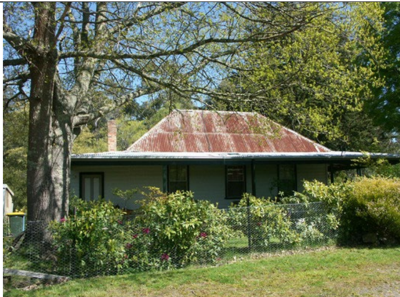
Photo 3: Dwelling, 4 Albert Street, Blackwood front (east) and south elevations, 2009.
