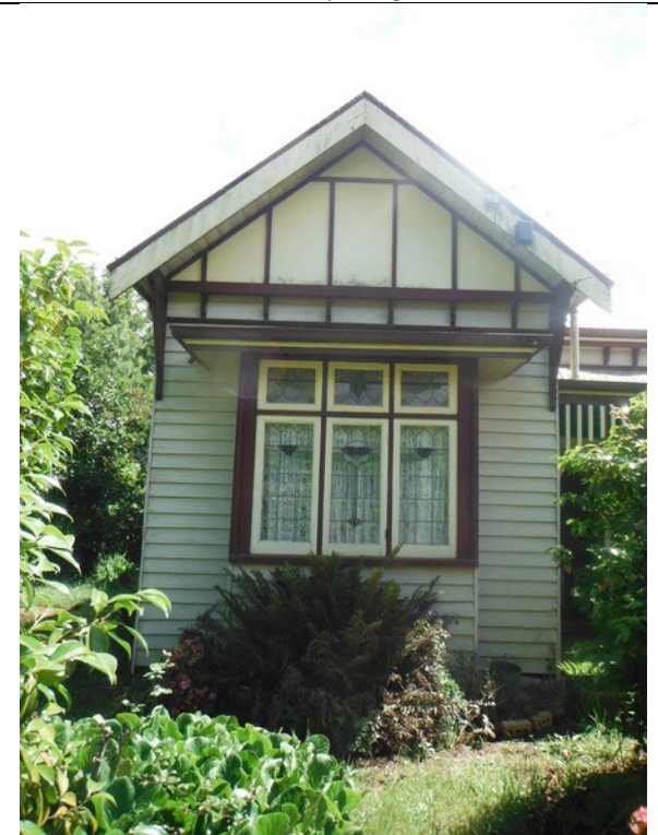
Photo 7: Sunny Rise, detail of front gable end, 2014. Source: Dennis Speilvogel.
