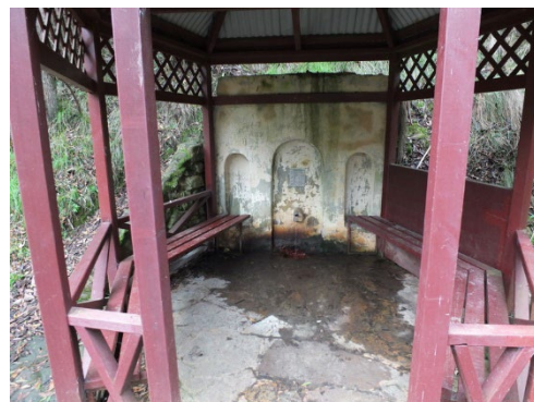
Photo 3: North Pavilion, 2014, showing the rendered masonry wall with water outlet.
