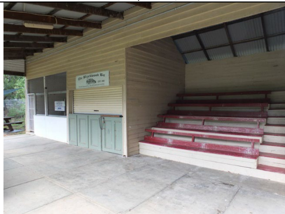
Photo 6: Detail of the east elevation of the timber pavilion, 2014.
