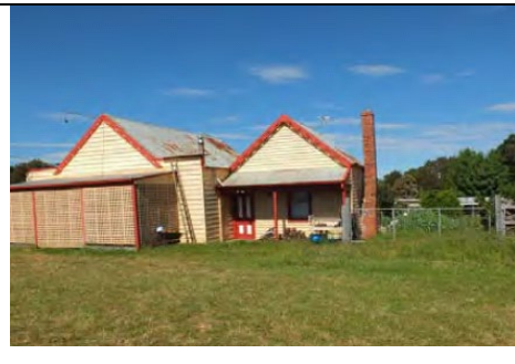
Photo 8: Dwelling & Former Store, 32 Russell Street, Gordon, 2014. Source: David Rowe.
