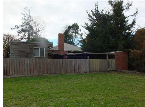
Photo 11: Brick Interwar Bungalow (Building 3), south elevation with rear early brick skillion outbuilding (right) and introduced timber outbuilding (left), 2014.
