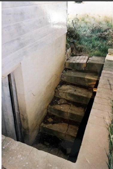
Photo 5: Former 'The Pines' dairy, steps detail, n.d. [c.1990s].
