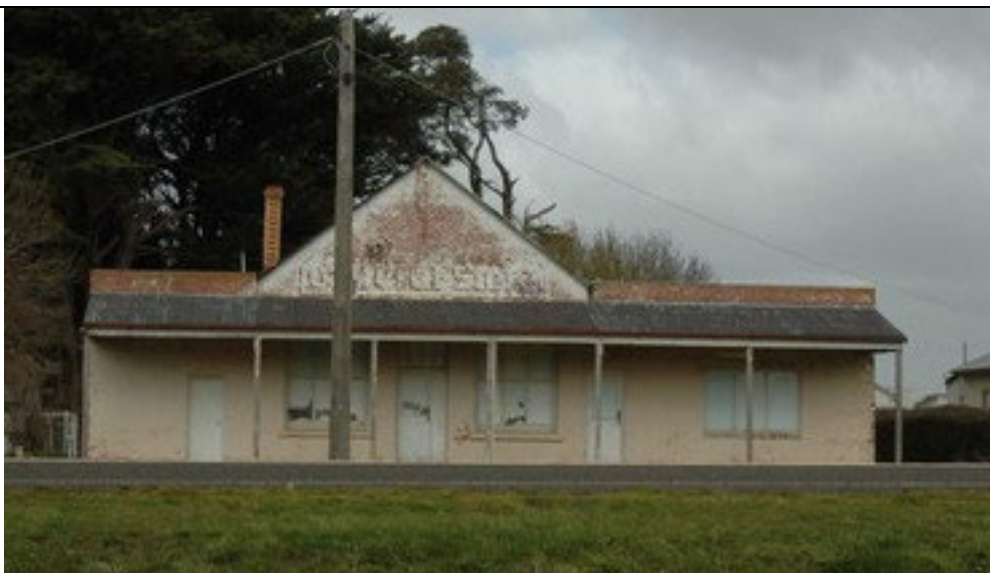
Photo 5: Former Store, 720 Bungaree Wallace Road, 2009 prior to the removal of the introduced overpainting.
