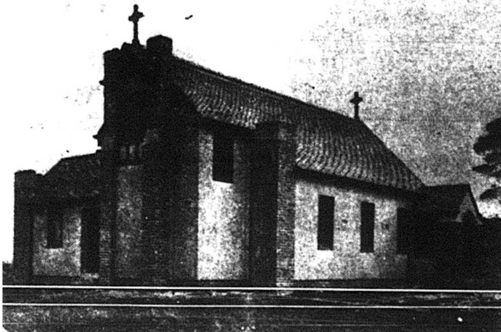
Photo 4: St. Mark's Church of England Church, Gordon, 1937.
