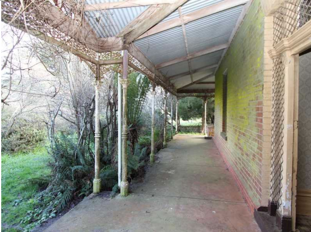
Photo 8: View under front verandah (looking west), 2012.
