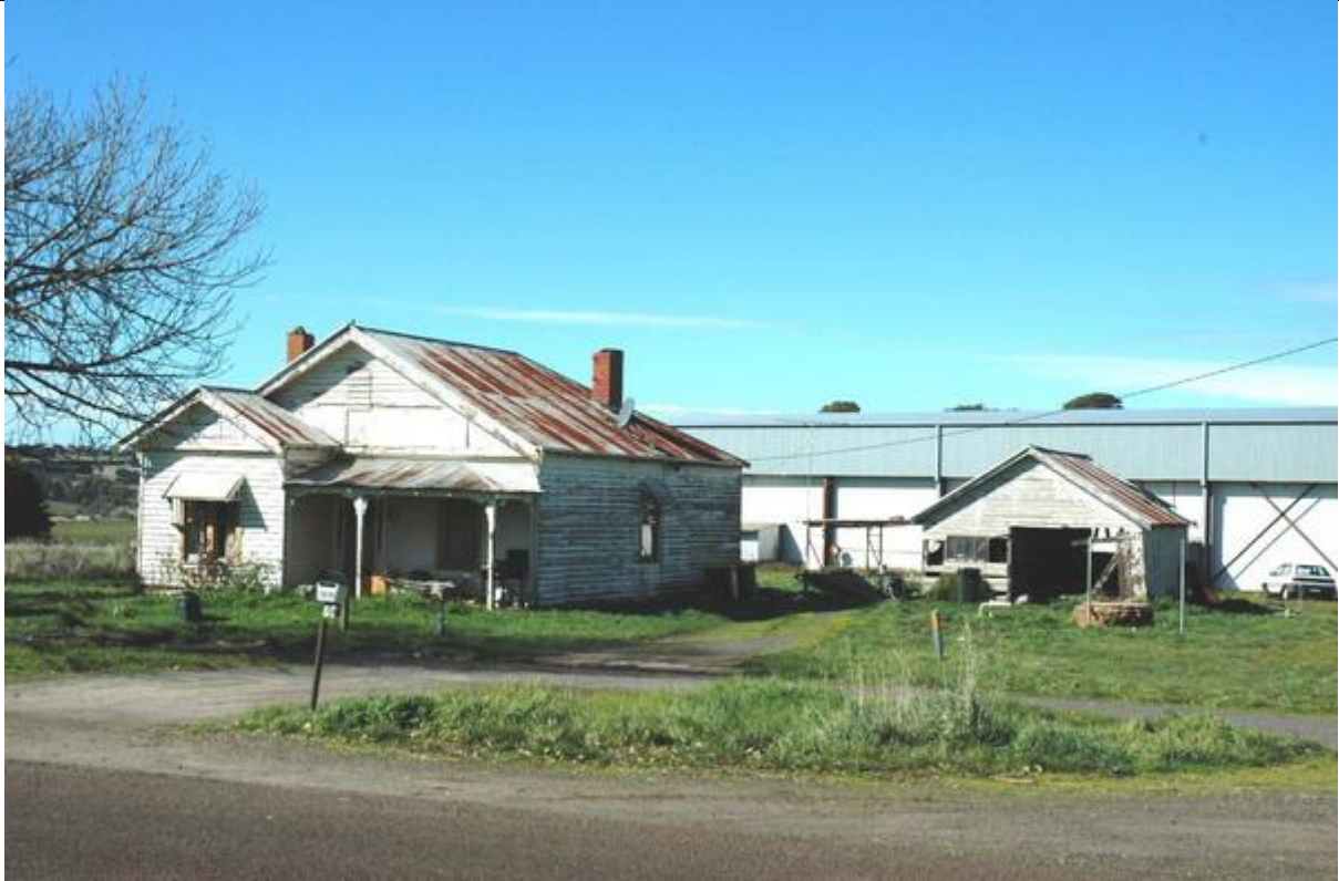
Photo 14: Timber Interwar Bungalow and gabled outbuilding, north and west elevations, 2009.
