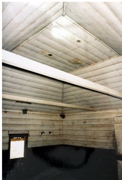
Photo 7: Former 'The Pines' dairy, interior, n.d. [c.1990s].
