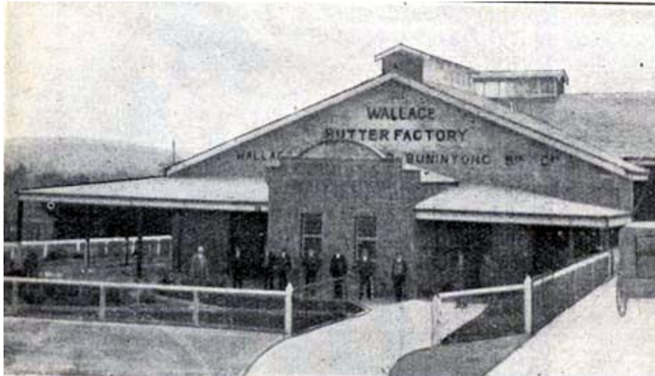
Photo 21: Butter factory, front elevation, showing the addition of the central parapeted bay at the front, c.1928.
