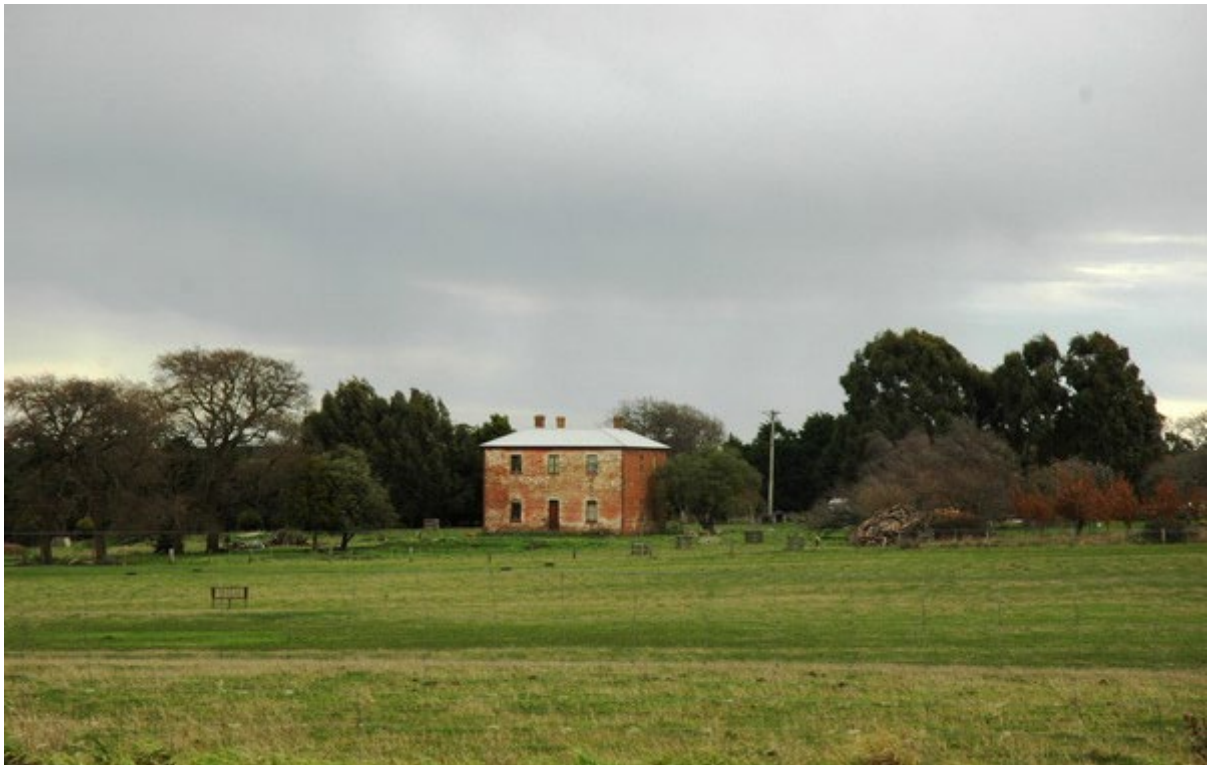
Photo 2: Oakvale front (east) elevation, viewed from Boundary Road, 2009.
