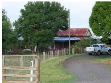
Photo 4: The Pines, 52 Sullivans Road, Millbrook, 2009.
