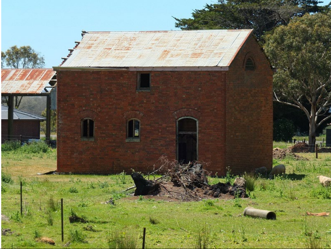
Photo 3: Former stables, 4 Erin Court, west and south elevations, 2014.
