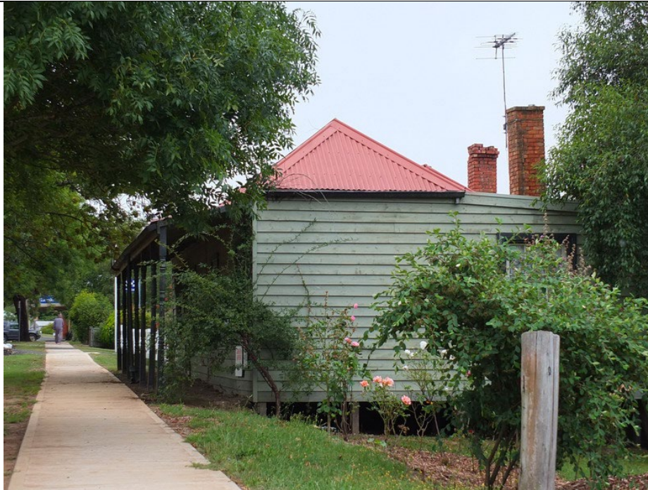
Photo 3: Dwelling and former bakery and store, east elevation showing replacement floor stumps and weatherboard wall cladding, as well as rear skillion addition, 2015.
