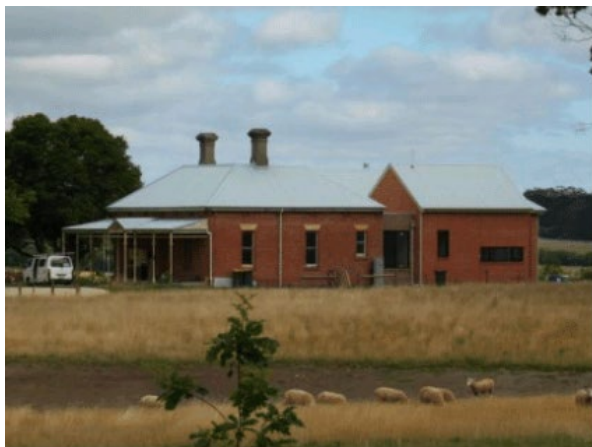
Photo 5: Former Ryan Family Farm, 91 Ryans Road, Millbrook, 2015.
