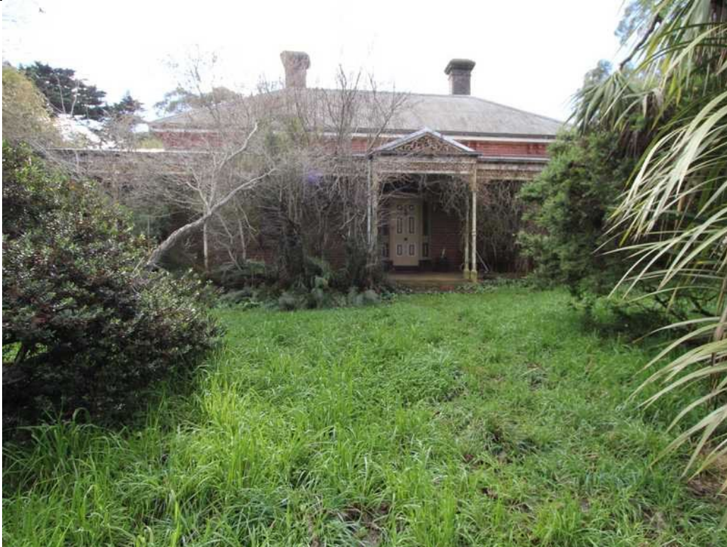
Photo 6: Front (south) elevation of main dwelling, 2012.
