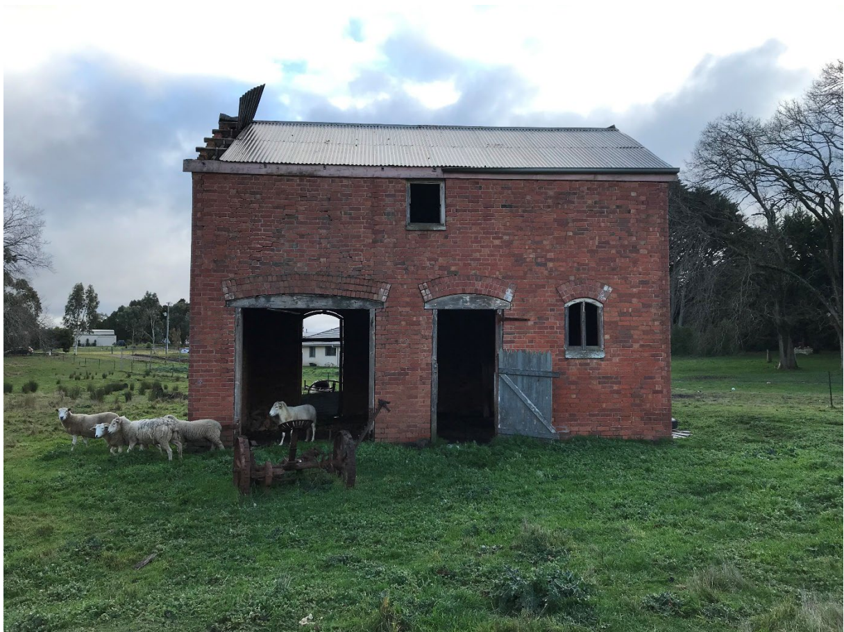
Photo 2: Former stables, 4 Erin Court, west elevation, 2020.
