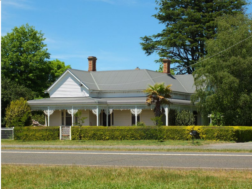
Photo 2: Dwelling, 720 Bungaree Wallace Road, front and side (west) elevations, 2014.
