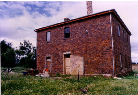
Photo 6: Oakvale, rear (west) elevation, 1998. Source: Wendy Jacobs
