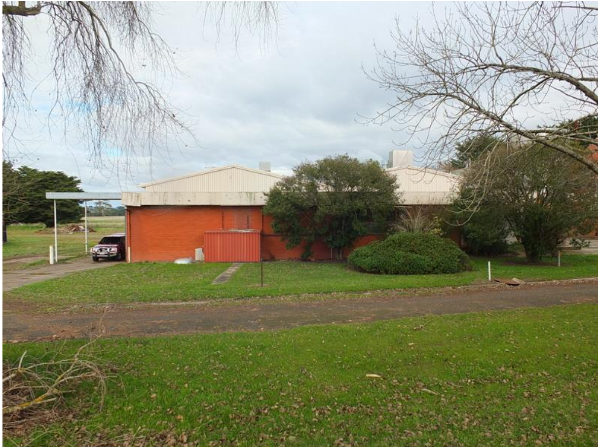
Photo 9: Former Cheese Factory (Building 2), north elevation, 2014.
