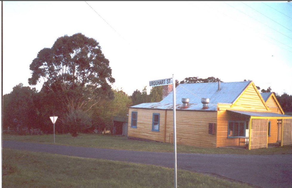
Photo 4: Dwelling and former Store, north and west elevations, 2002.
