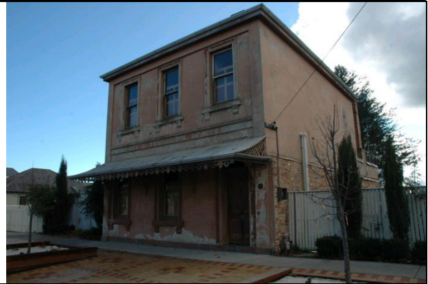
Photo 10: Former Post and Telegraph Office, 140 Inglis Street, Ballan, 2010.
