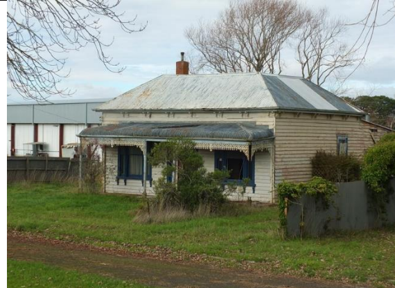
Photo 13: Late Victorian timber dwelling (Building 5), north and west elevations, 2014.
