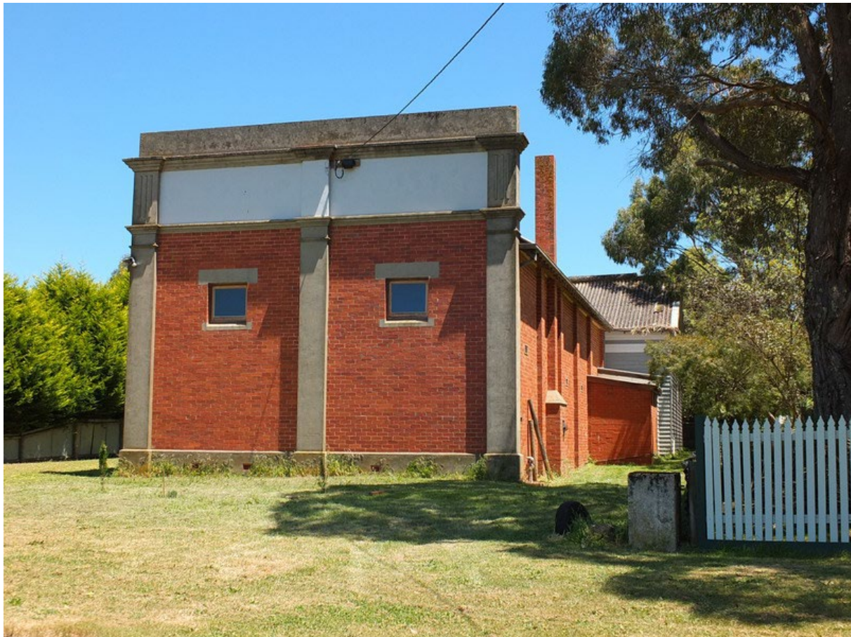
Photo 2: Masonic Temple, front (east) and side (north) elevations, 2014.
