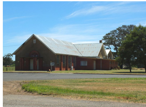
Photo 4: former Mechanics Institute and Free Library building (c.1928 with c.1958 additions), at 221 Bungaree-Wallace Road Bungaree, Source: David Rowe and Wendy Jacobs.
