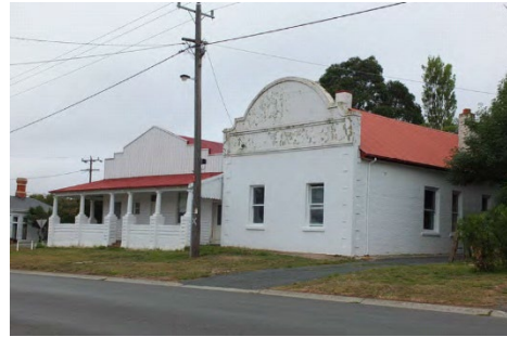
Photo 10: Former Williams Hotel, 69 Main Street, Gordon, 2015. Source: David Rowe.
