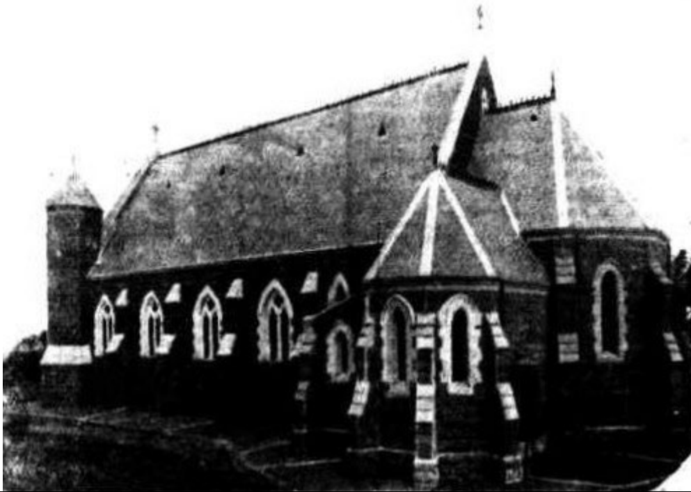
Photo 7: St. Patrick's Church showing sanctuary and sacristy additions, 1912.
