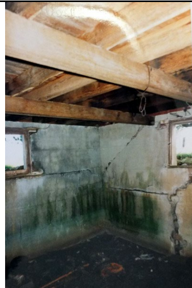
Photo 6: Former 'The Pines' dairy, basement interior, n.d. [c.1990s].
