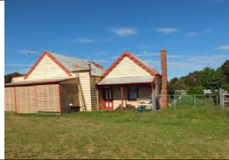
Photo 6: Dwelling & Former Store, 32 Russell Street, Gordon, 2014. Source: David Rowe.
