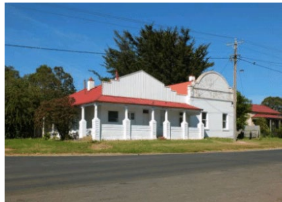
Photo 5: Former Williams Hotel, 69 Main Street, Gordon, 2014. Source: David Rowe.
