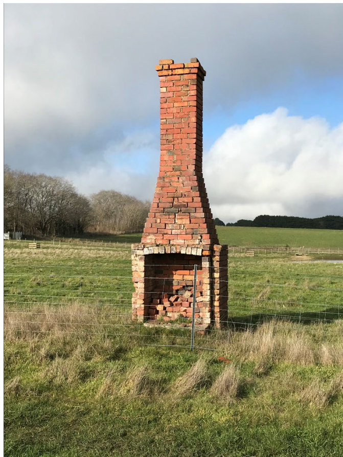
Photo 9: Chimney stack from shearer's quarters, July 2020
