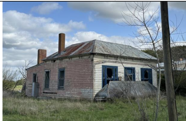
Photo 14: Late Victorian timber dwelling (Building 5), north and east elevations, 2024.
