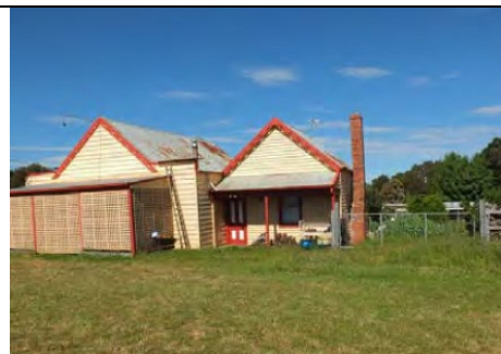
Photo 7: Dwelling & Former Store, 32 Russell Street, Gordon 2014. Source: David Rowe.
