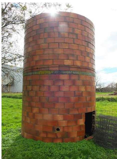
Photo 15: Terra cotta tank, south and east elevations, 2014.
