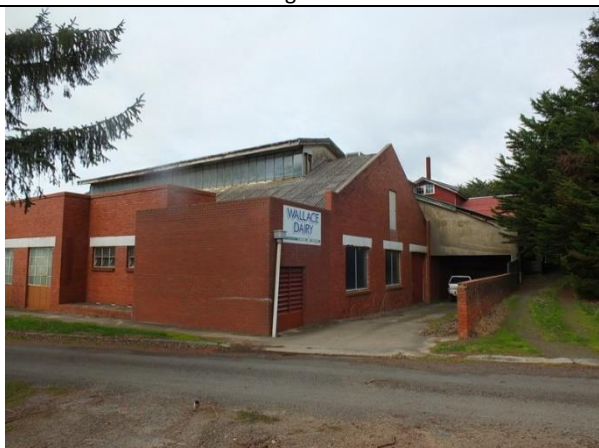
Photo 7: Former Butter Factory (Building 1), north elevation, 2014, showing the additions of the 1940s-50s at the front.
