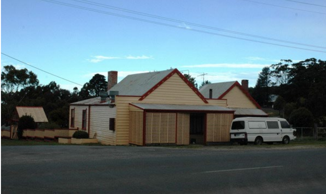
Photo 3: Dwelling and former Store, north and west elevations, 2009.
