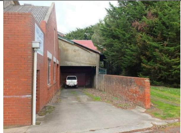
Photo 4: Former Butter Factory (Building 1), north elevation (west end), 2014. The projecting gable end represents the addition of 1922. The roof projecting above is the gambrel-roofed porte-cochere of 1908.
