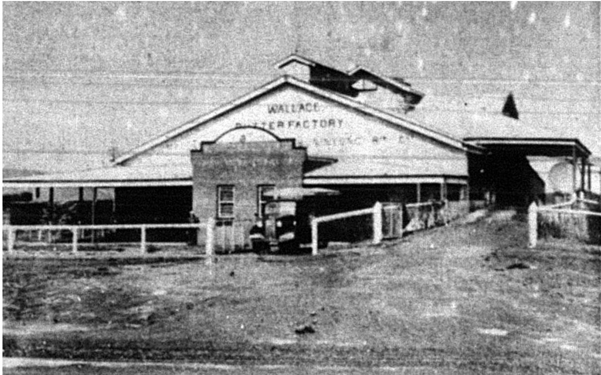
Photo 22: Butter factory, front elevation, showing two storey gabled attic addition behind the monitor light of the front gabled wing), 1939.
