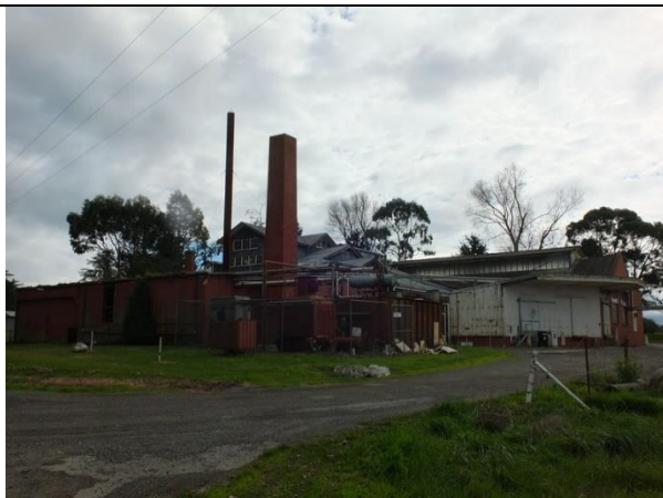
Photo 5: Former Butter Factory, south and east elevations, 2014. The elevated gabled wing behind the chimney stack is the addition of the 1930s, the lower portions (including the lower gabled form on the right side) being the original building of 1908.
