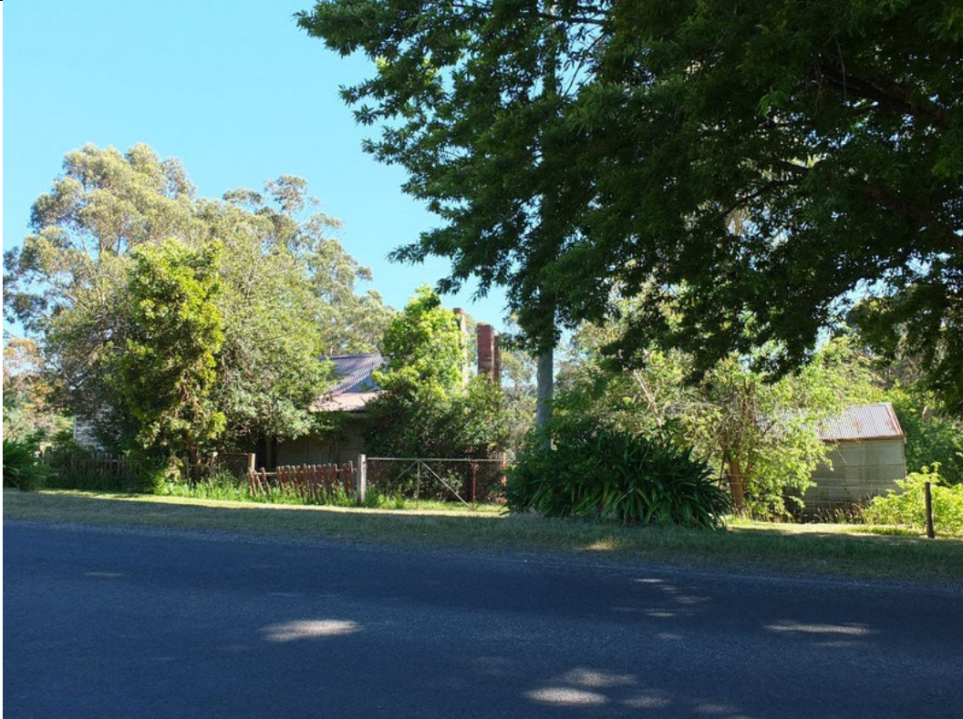
Photo 2: Dwelling, 56-60 Main Street, with outbuilding on the right, 2014.
