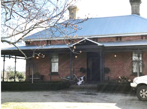
Photo 2: façade of dwelling, July 2020
