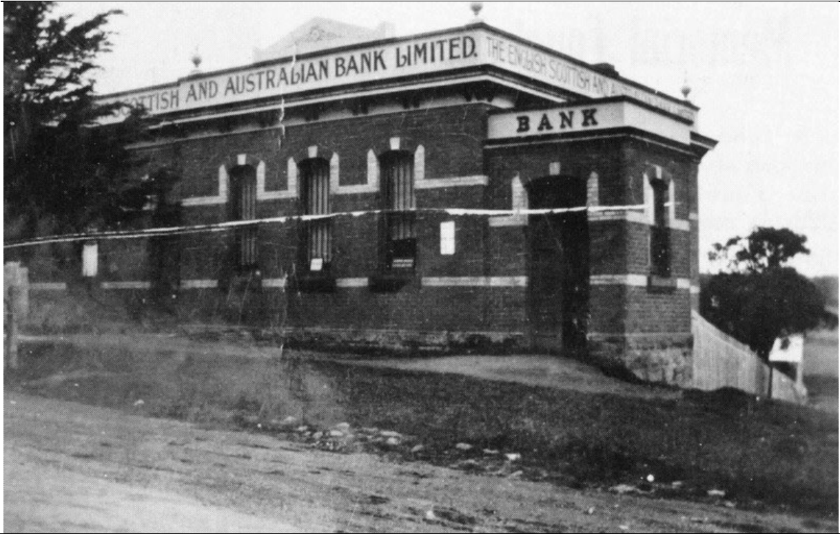
Photo 6: Former London Chartered Bank (when the ES & A Bank), n.d. [c.1930], 64 Main Street, Gordon.
