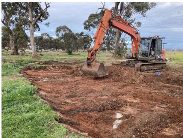
Figure 1: Remediation excavation showing undisturbed natural soil at the excavation base.
