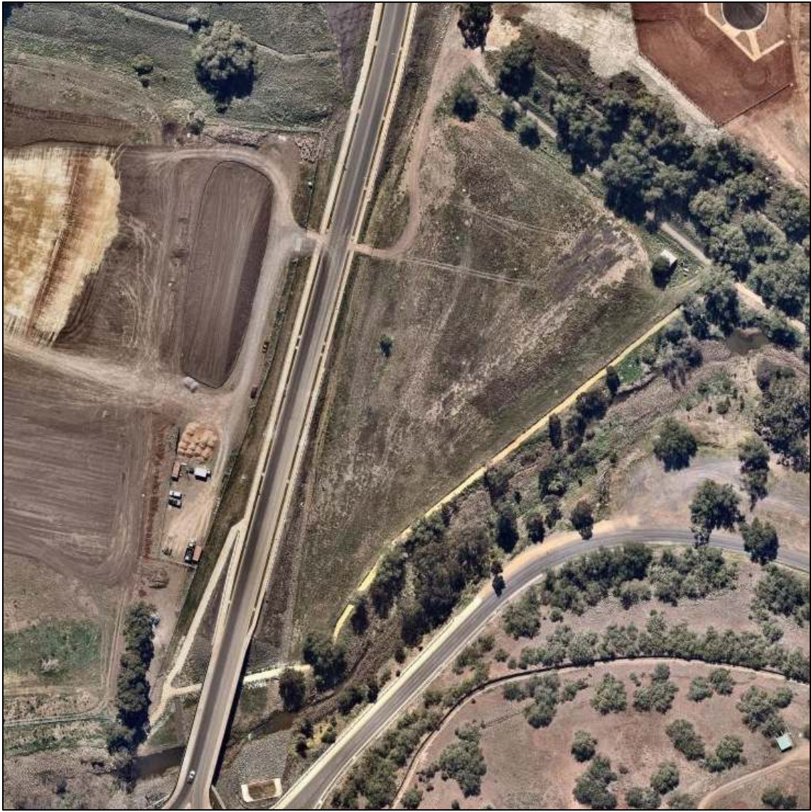
Figure 7: September 2018 Nearmap aerial image of the study area
