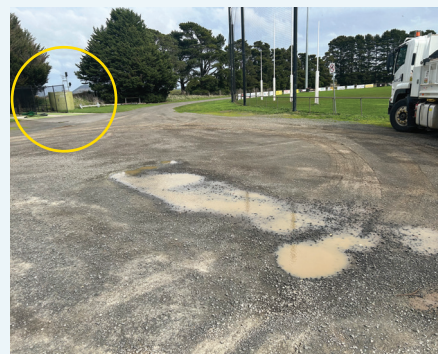
Site of cricket nets highlighting the runoff across the gravel road surface
