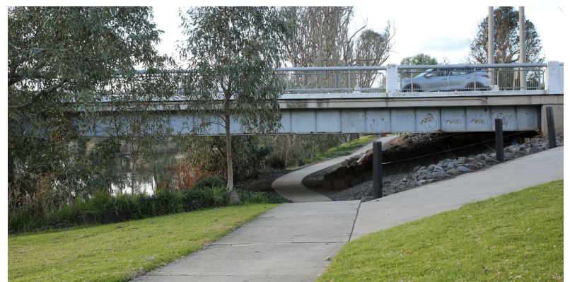
Figure 18: Example of a river path under a major road: Calder Highway at Bridgewater on Loddon
