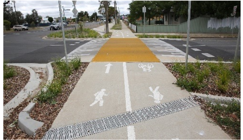
Figure 17: A Safe System "Bend In" priority raised crossing for shared paths (Ballarat)
