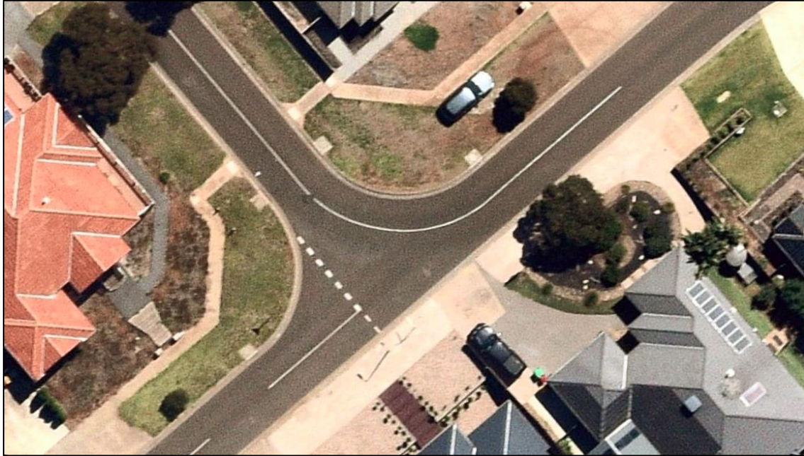
Figure 5 Example of a modified T-intersection (from Nearmap aerial photography)
