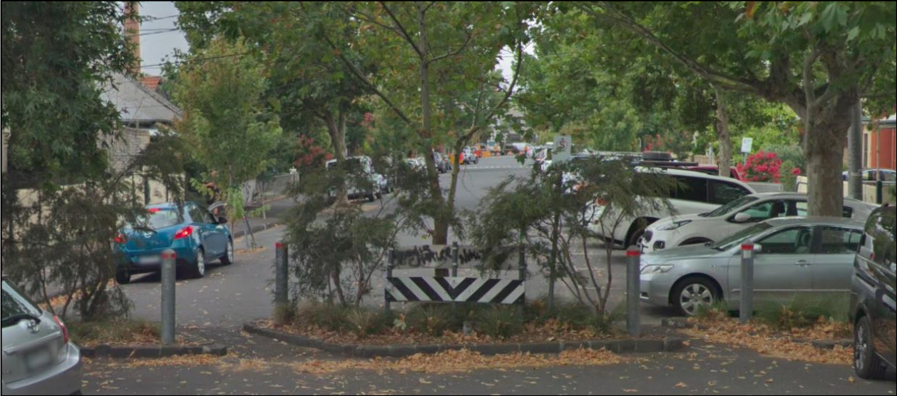
Figure 10 Example of a full road closure (from Google Maps Streetview)
